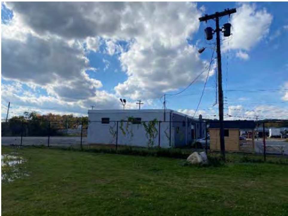
Industrial/commercial building along the southern portion of the Site.
