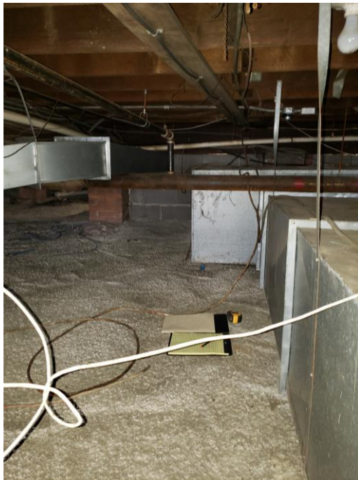
View Toward Machinery Room
