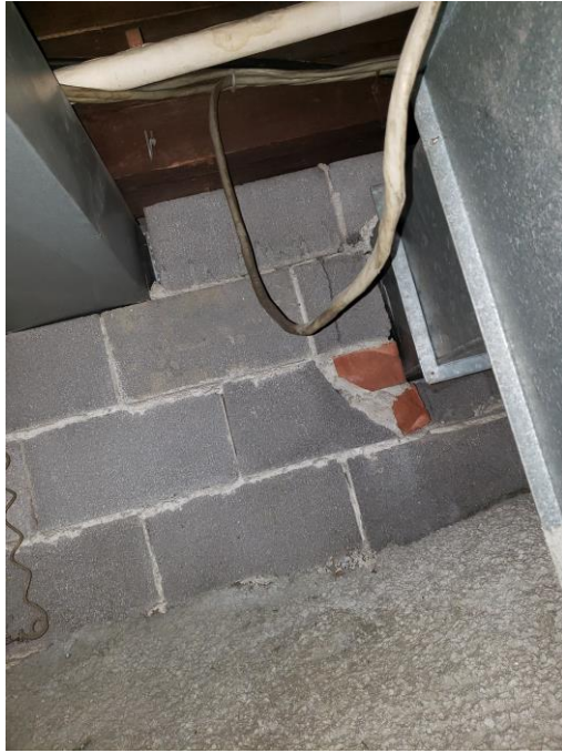
Penetrations into Machinery Room
